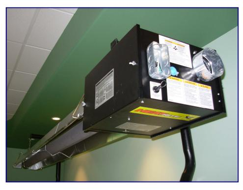
Radiant tube heating offers a convenient and effective alternative to standard brooders. Ceiling mounting provides wide even coverage in the barn.
